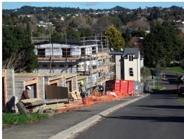
New intensive housing built in Woodglen area (2010)
