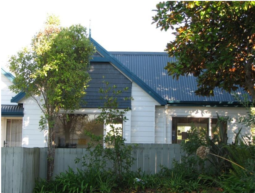
Car Park View of Unit 1, 298 West Coast Rd
